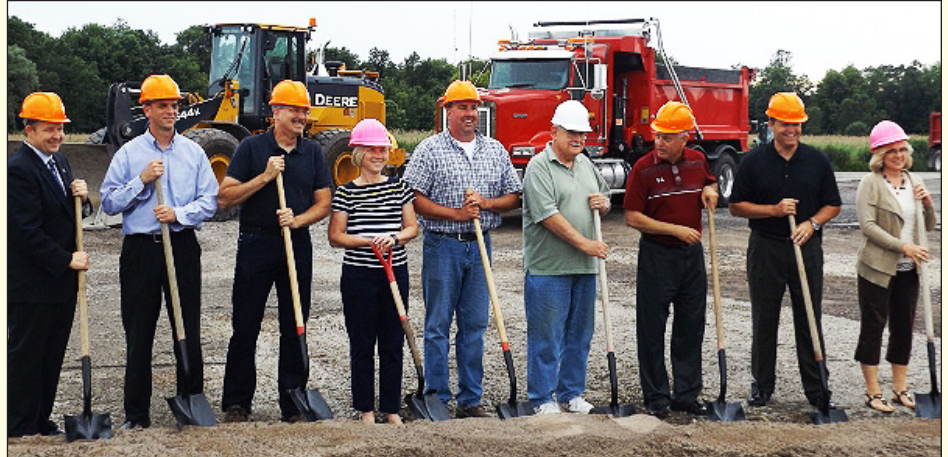
Groundbreaking for the new highway garage was held in June 2017. Pictured, from left, are: Town Manager Doug Finch; Scott Bova, AIA, MRB Group (the Town's consulting engineering firm); Town Board member Kevin Reynolds; Town Board member Linda Dworczyk; Highway Superintendent Jim Fletcher; Town Board member Terry Fennelly; Supervisor Greg Westbrook; Deputy Supervisor Keith Cutri; and Town Clerk Jean Chrisman.
