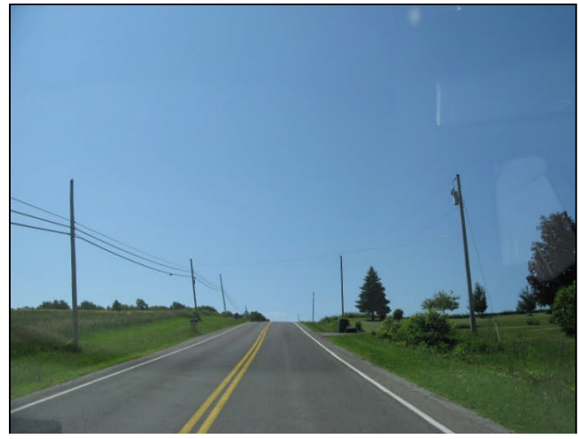
Aerial Utility Lines along Brickyard Road
