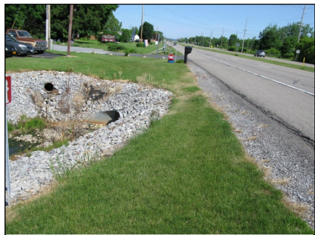
Existing stormwater management facility will require modification to accommodate the trail
