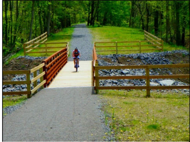
Auburn Trail Bridge over Irondequoit Creek
