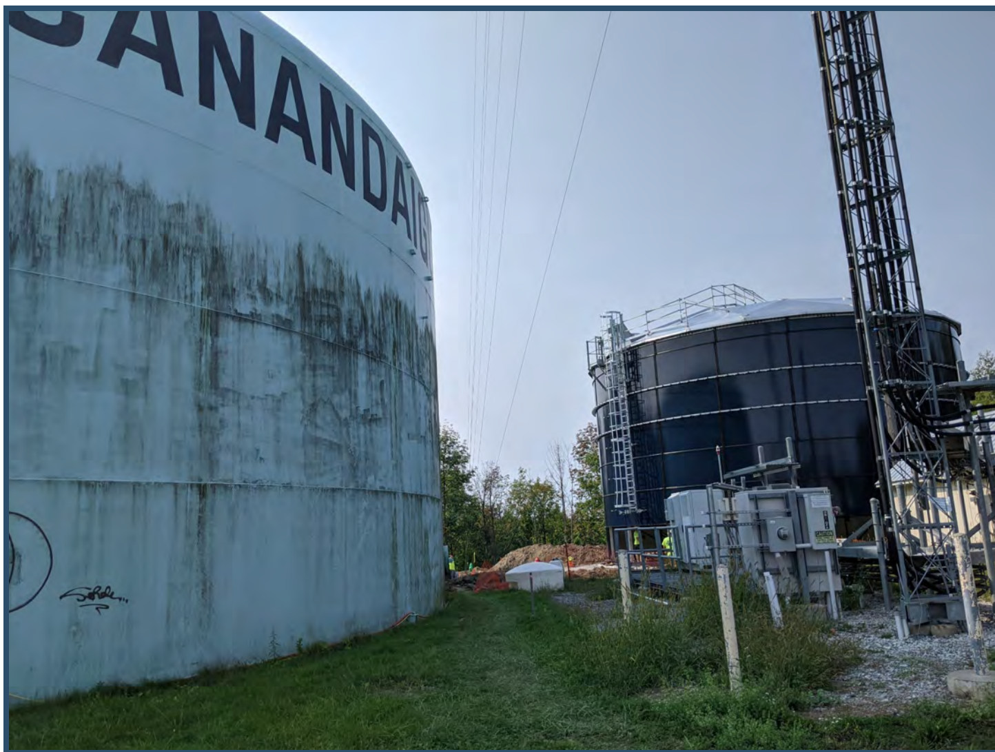
Raising the new water tanks in Cheshire, 2020.
