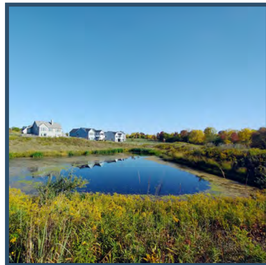
Stormwater Facility at Lakewood Meadows
