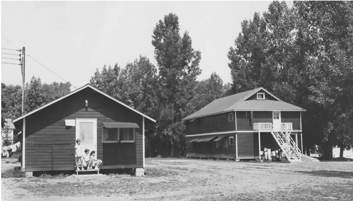
Figure 50. Two camp buildings at Camp Onanda. Source: West Lake Legacy .
