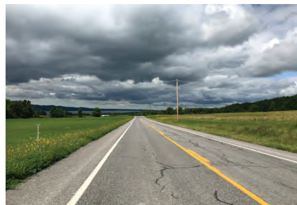
A Low traffic volume, wide shoulder, good pavement, no parking
