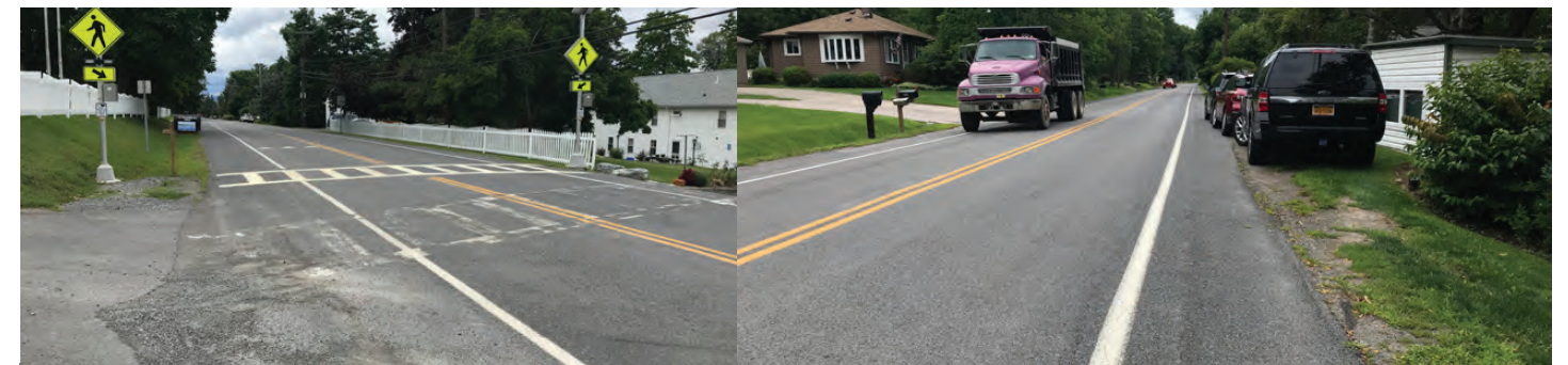
Le Tourneau Existing Enhanced Crosswalk
