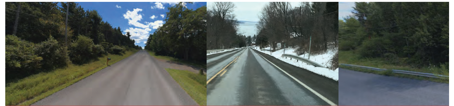
Typical View of Roadway with Driveways
