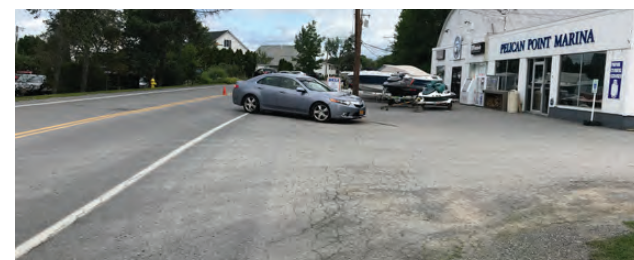
CR 11 at Pelican Point Marina
