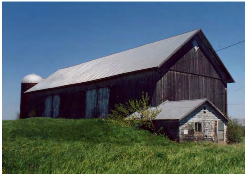
PHOTO 11: HAY BARN OWNED BY DAVID SAUTER, WEST AVENUE EXT. PHOTO CREDIT: RAY HENRY, TOWN HISTORIAN
