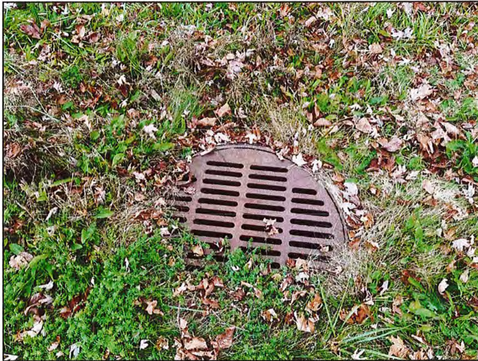
Photograph 13. Existing drainage on the western boundary of the APE, looking down.
