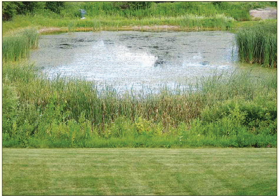
This is a good example of the natural buffer between the mowed lawn and the stormwater pond at one of the ponds at the Fox Ridge Subdivision in the Town of Canandaigua.
