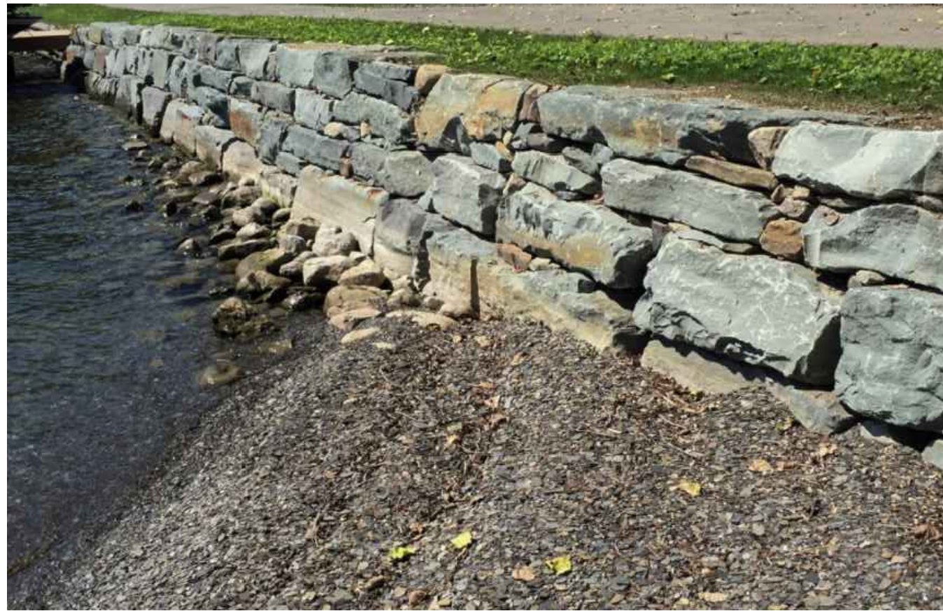
LIMESTONE RETAINING WALL EXAMPLE:
