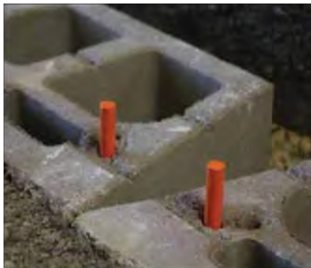
Diagram 5 - Pin Placement
