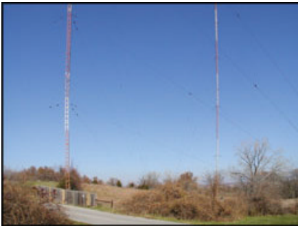
Physical changes in the antenna system can affect a directional array, but it is equally important to inspect tower fences and clear around vegetation
