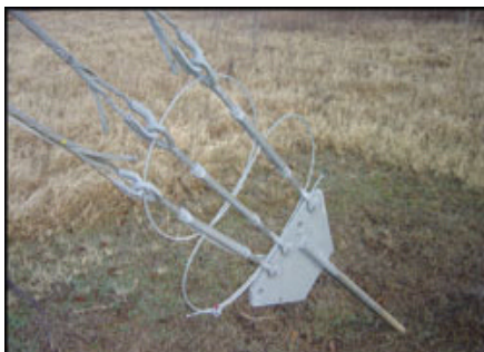
Guy anchor showing the turnbuckle safety in figure-eight formation as required by TIA/EIA 222.
