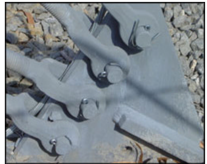
Stainless steel cotter pins are best. This anchor plate is cold galvanized for protection from rust.
