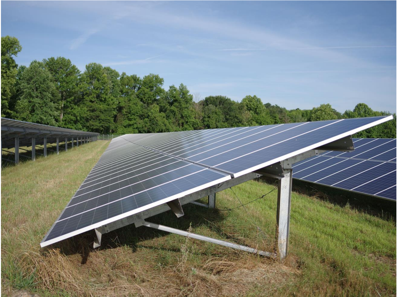
Photo 8: Fixed-Tilt Racking System
