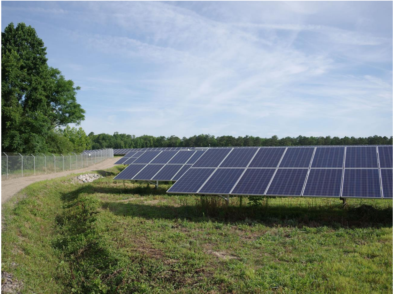
Photo 3: Ground-Mounted PV Modules, Diversion Swale, Perimeter Access Road, and Security Fence
