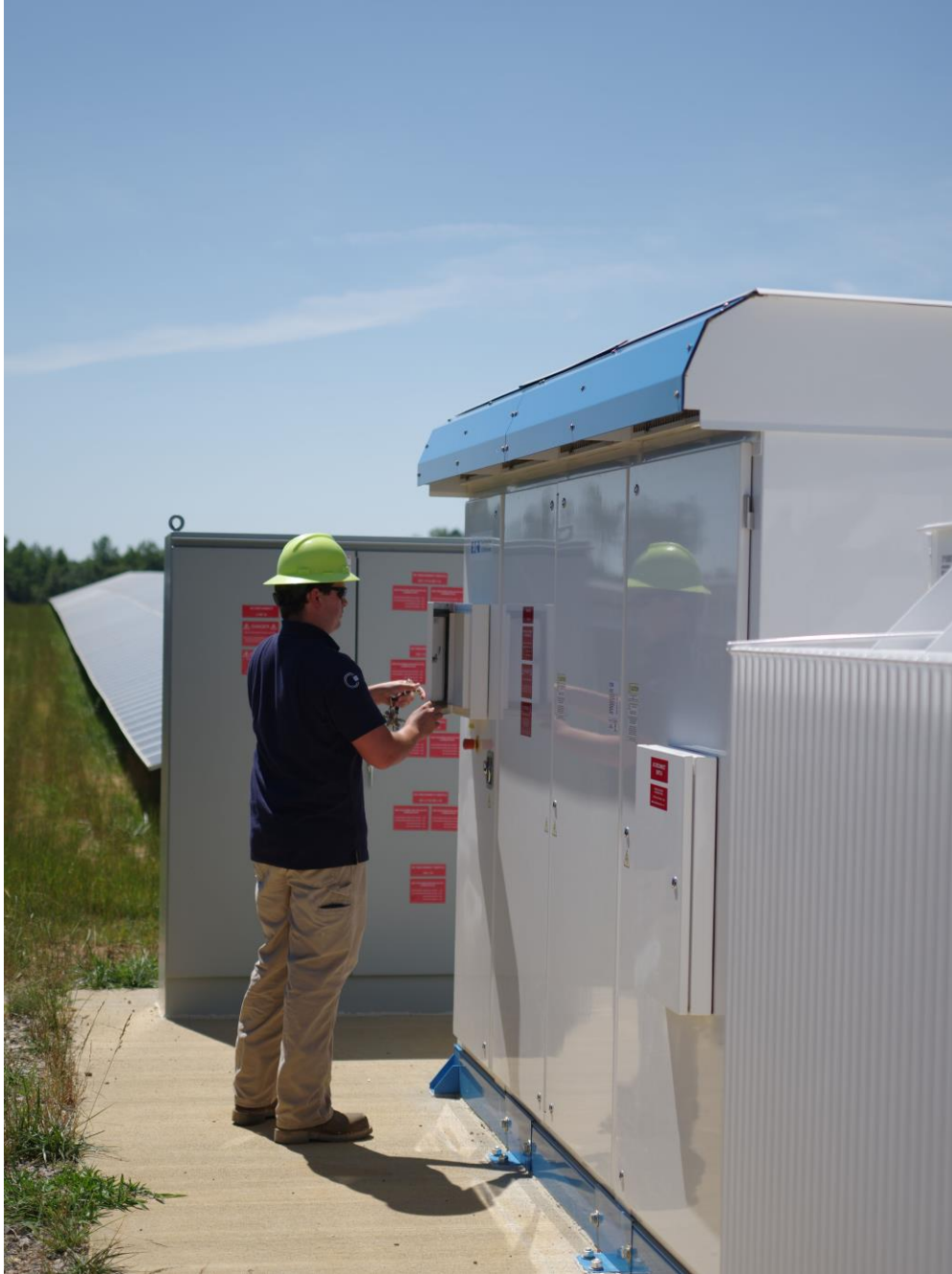
Photo 5: Central Inverter Height, as Compared to Average Human
