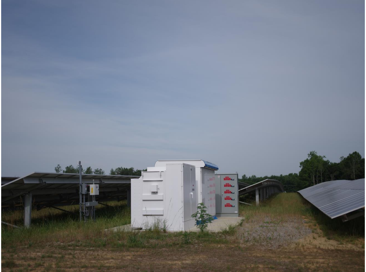
Photo 4: Central Inverter & Equipment Pad
