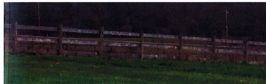
TYPICAL 4ft WOOD 3 PLANK FENCE to MATCH EXISTING LOCATED ON FIELD SIDE OF SOLAR ARRAY 4ft WIRE MESH 6X6 LIVESTOCK FENCE ON WOODS BACK SIDE
