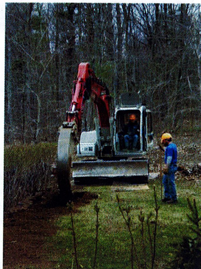
Trenching to break grafted roots
