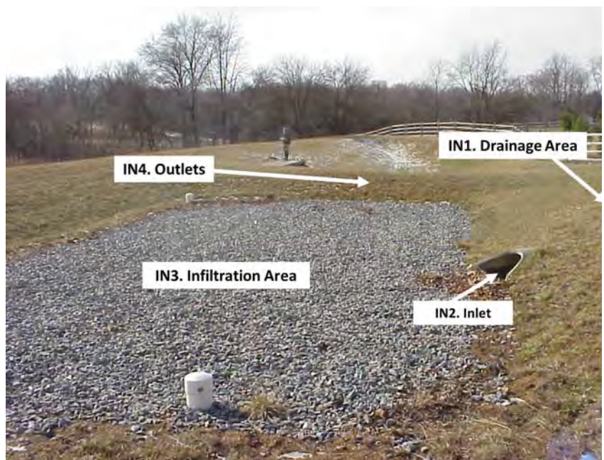
Figure 2.11.1 Key Areas for Level 1 Inspection of Infiltration Practice
