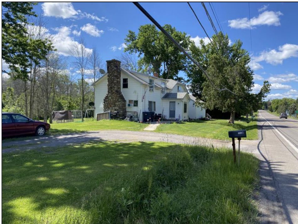
Photograph 28. House # 3555 NY Route 364 (East Lake Road), west of the APE, looking south / southeast
